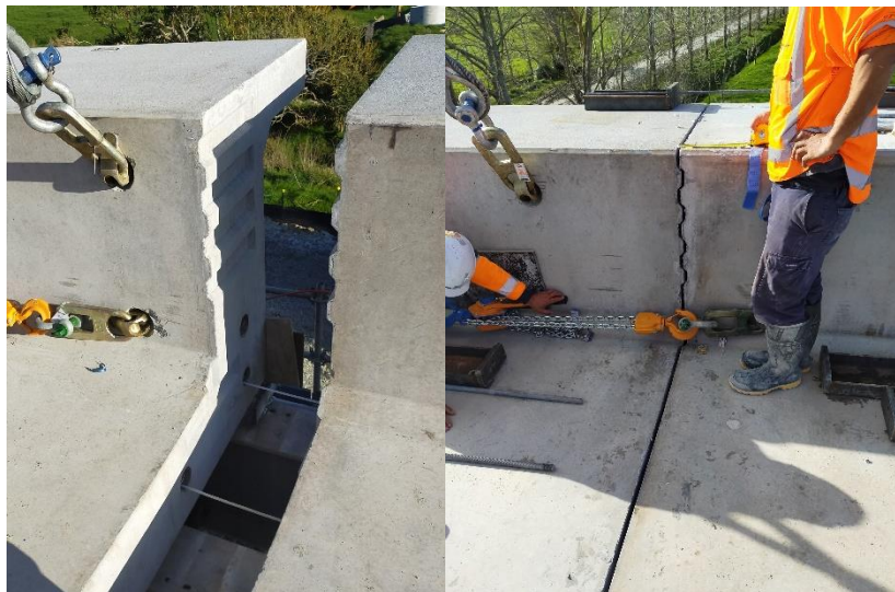
Figure 6. Trial fitment of segments at Bridge 126 NAL
