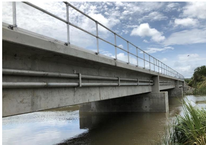
Figure 8. New Bridge 88 NAL
