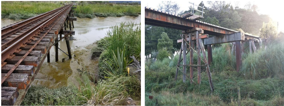
Figure 2. Bridge 89 and Bridge 100 NAL before replacement
