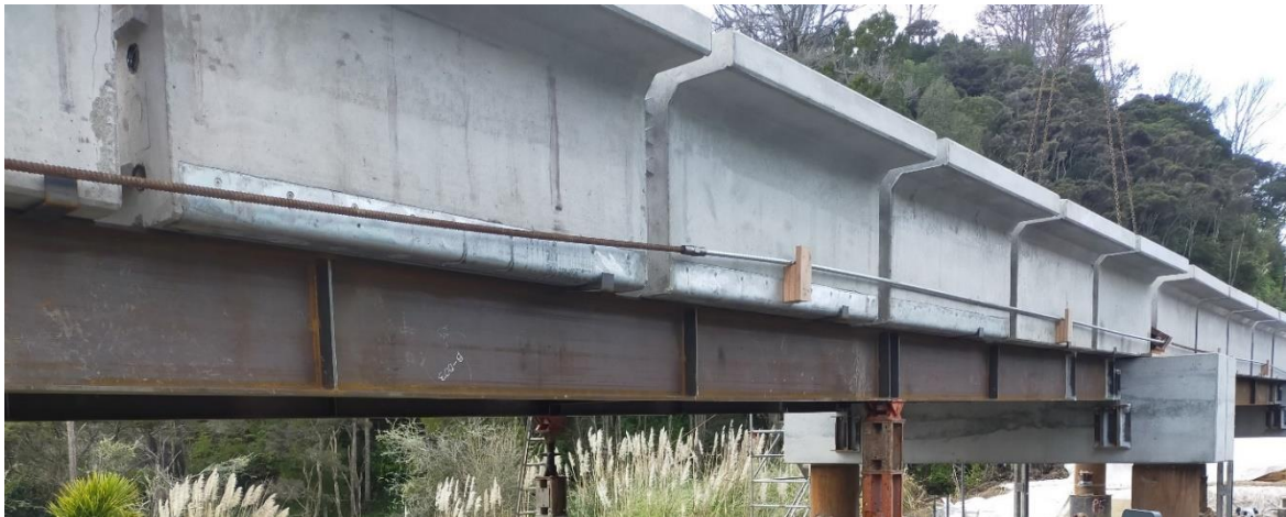
Figure 5. Precast segments supported on temporary works at Bridge 100 NAL
