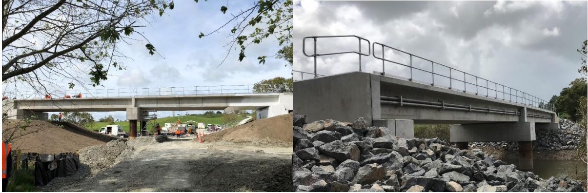
Figure 9. Bridge 126 NAL near completion and Bridge 168 NAL
