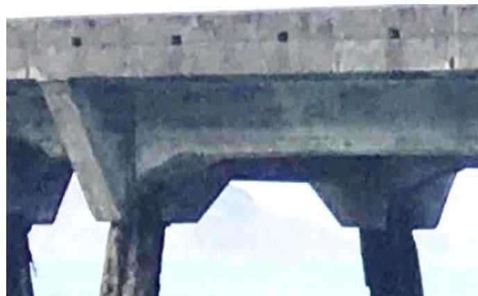
Figure 2. Photograph Showing Profile of the Headstocks and Longitudinal Beams
