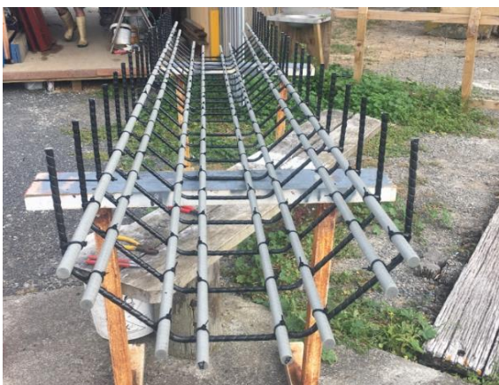
Figure 4. FRP Reinforcement Cage Half
