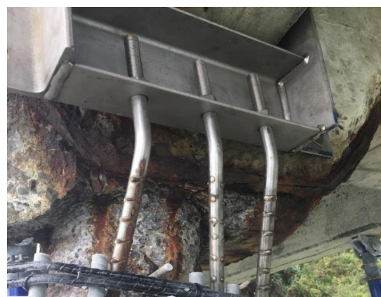
Figure 5. Starter Bar Connection
