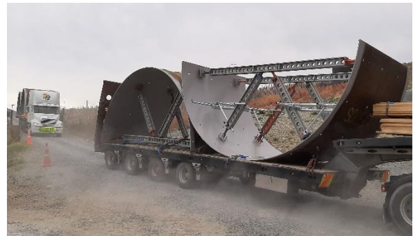
Figure 7: Tunnel liners arriving on site
