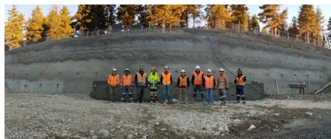
Figure 3: Completion of 6m high retaining wall
