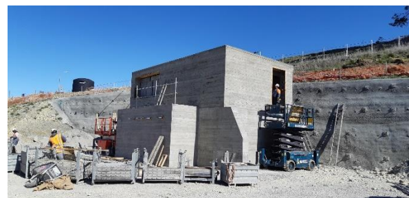
Figure 12: Control room structure
