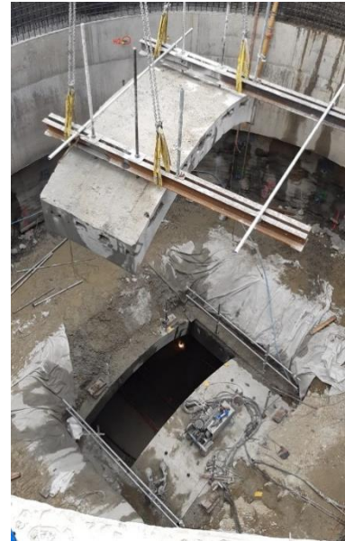
Figure 6: Removal of tunnel crown for access
