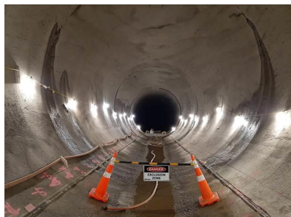
Figure 5: View inside the existing tunnel
