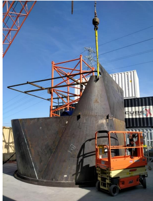
Figure 8: Fabrication of stent underway in vertical position
