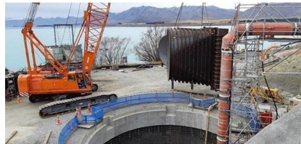
Figure 9: Installing the Stent in two halves
