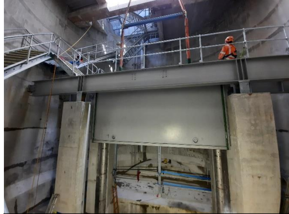
Figure 13: Gate installation
