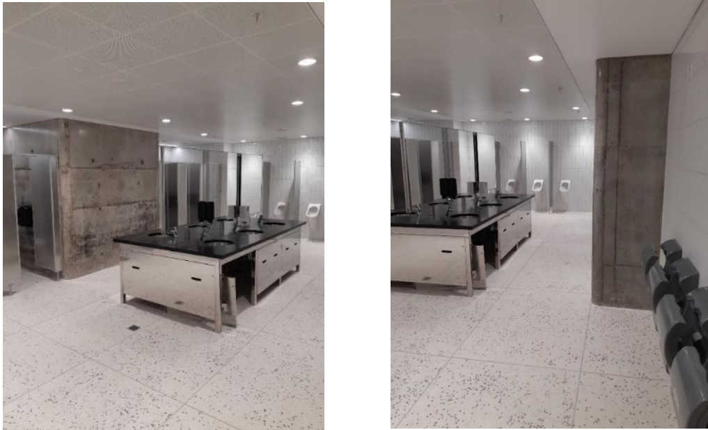
Figure 20: CPO Columns exposed concrete appeal inside public toilets at B1 level
