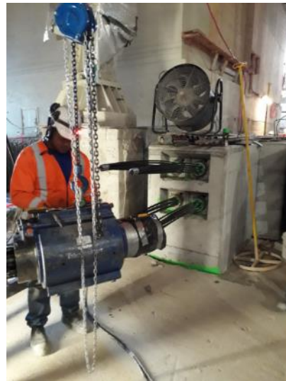
Figure 11: Concrete underpinning reinforcing and PT ducts through structures (left) Post tensioning works (right)
