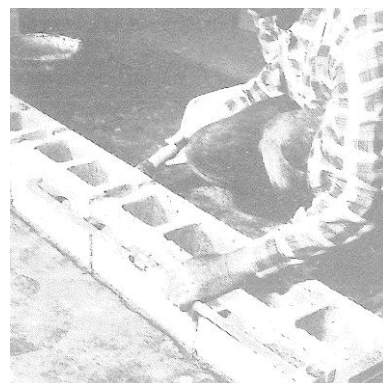
Figure 9 Check alignment
