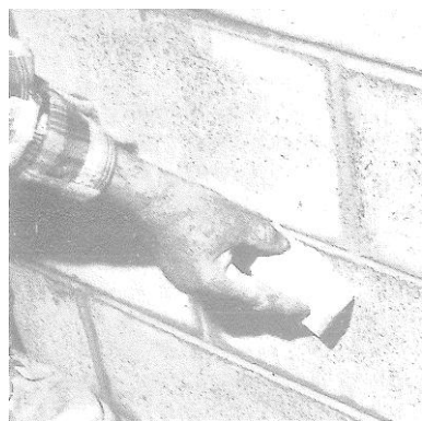
Figure 31 Rub with concrete block
