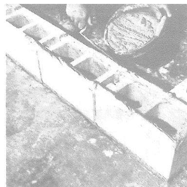
Figure 12 Face shell mortar bedding
