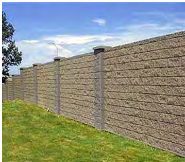
Figure 3: Split Block Wall (Image Source: http://www.blockwall.org/ )
