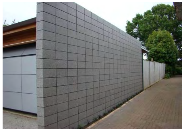
Figure 3: Coloured Honed Blockwork
