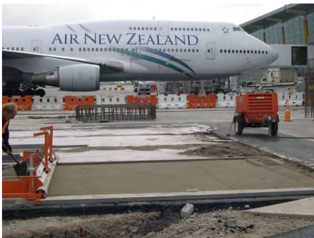
Figure 30: Christchurch Airport Apron Slab 80 mm Pavers
