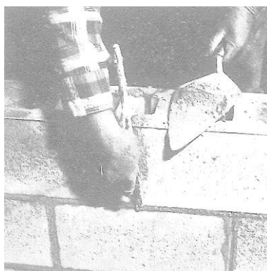
Figure 26 Packing vertical joint
