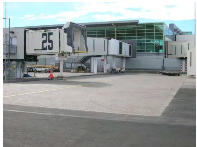
Figure 31: Christchurch Airport Apron Slab 80 mm Pavers
