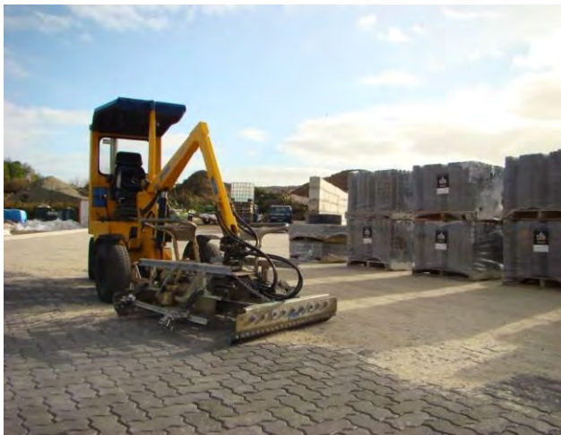
Figure 28: Paver Laying Machine
