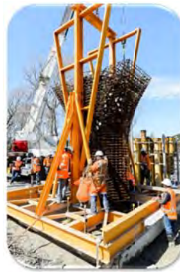
Cage lowered to final position
