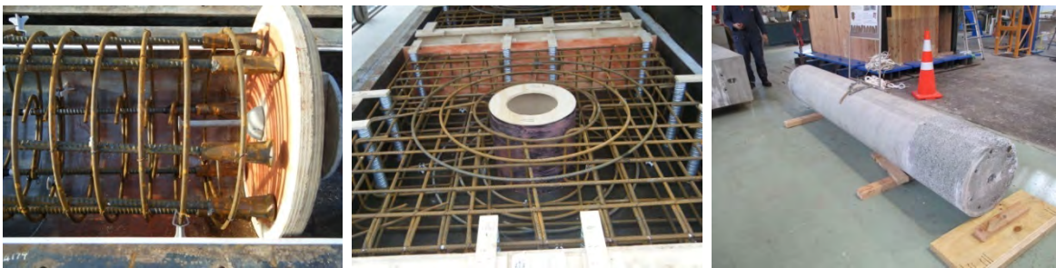
Figure 5. (Left) Foot inserts for column rebars, (Middle) Circular reinforcement around the socket, (Right) Column with roughened surface
