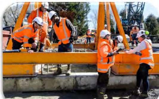
Column cage plunge frame setup
