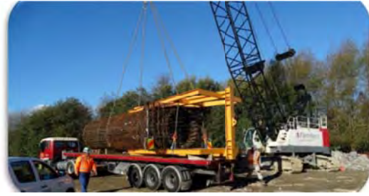
Column cage delivery
