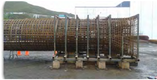
Column cage fabrication in the Jig
