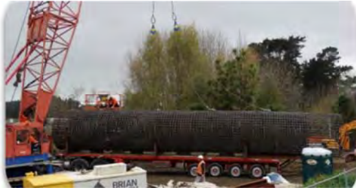
3m pile cage delivery
