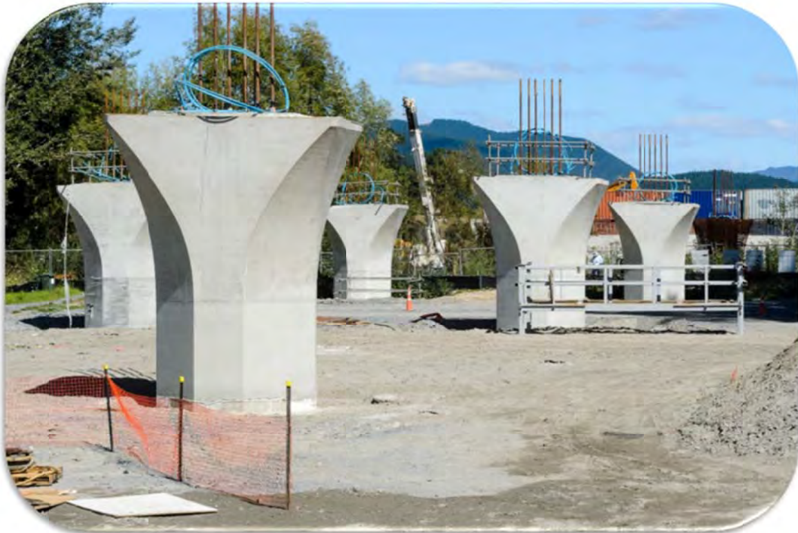
Figure 18: Completed columns for hammered-head piers of Waikanae River Bridge
