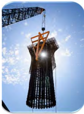
Column cage lifting and slewing
