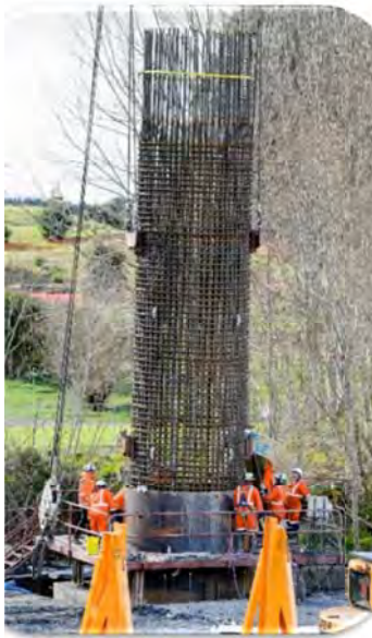
3m pile cage installation
