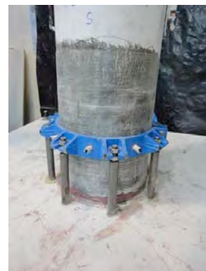
Figure 5c. Column after repair
