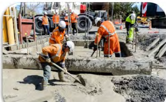
Top of pile clean up
