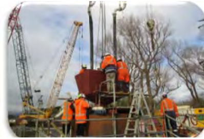
Concrete pour using specially designed hopper
