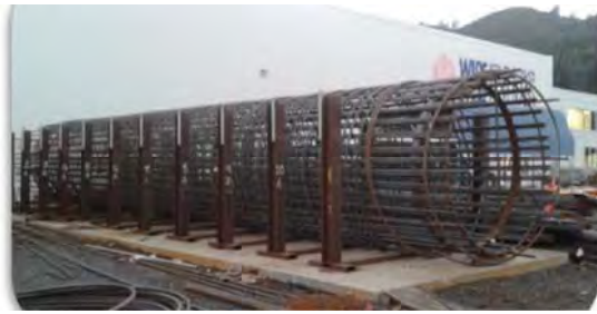
3m pile cage fabrication
