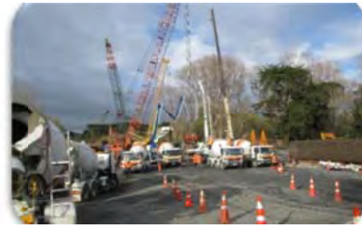
Concrete pour set up with two pumps
