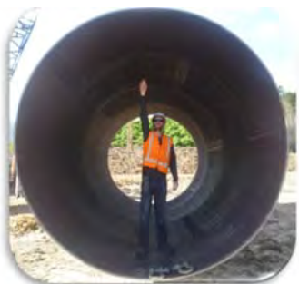
3m Temporary steel casing
