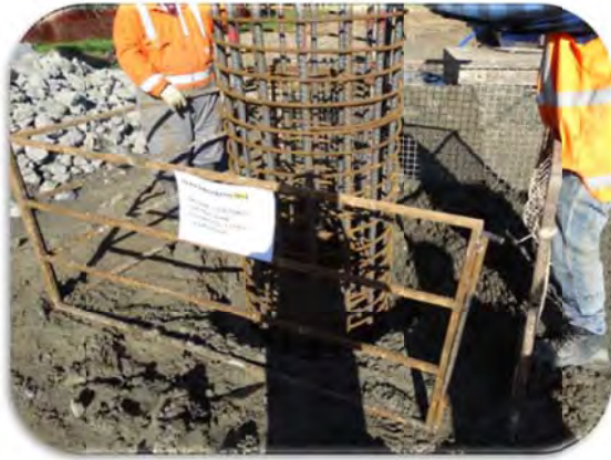
Figure 15: A dummy cage plunging trial in concrete to measure the initial set time of concrete and cage plunging ability with the time
