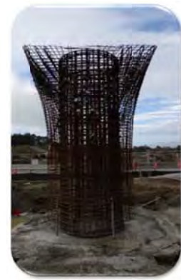
Plunged column cage after removal of temporary frame
