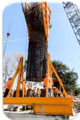
Column cage introduced into plunge frame
