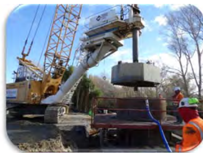
3m pile drilling with Liebherr 885 and RT3 Table mount Rig
