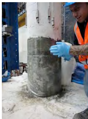
Figure 5b. Application of FRP
