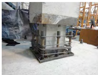
Figure 9b. Placement of column
