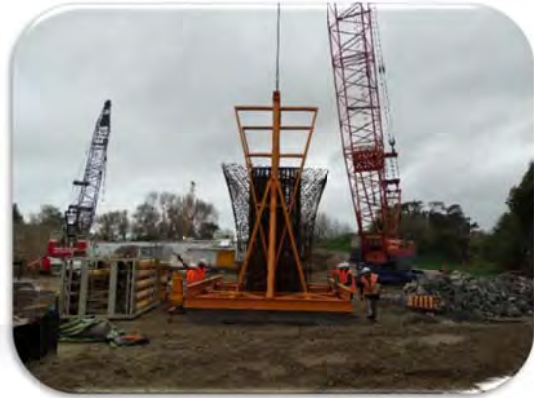
Figure 16: Lifting frame and column cage plunging trial to measure the total time of plunging operation
