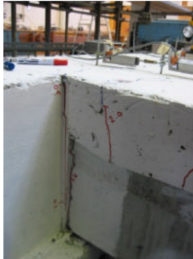
Figure 5-15. Photo showing the residual crack width at -2.0% (-1.85%) drift.
