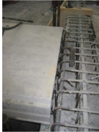
(b) Unit being positioned
