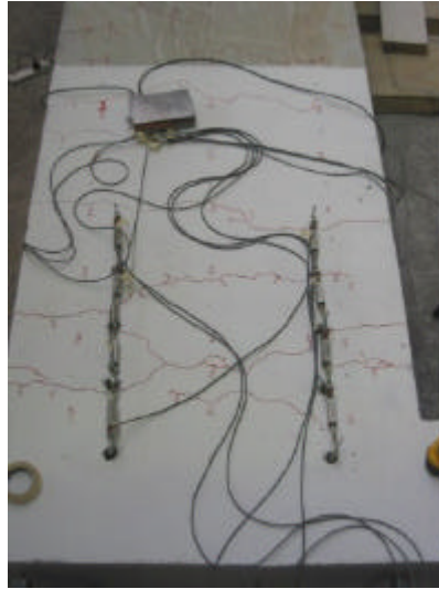
Figure 5-25. Cracks that had formed within the topping at -1.0% (-0.76%) drift.
