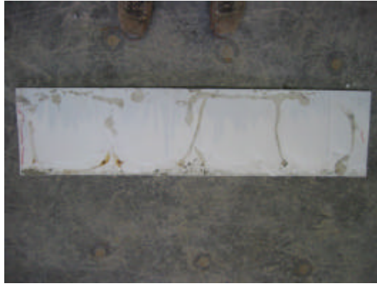
Figure 7-1. Grout seepage into the compressible backing board.
