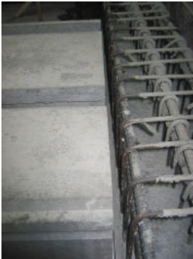
(c) Unit in place
