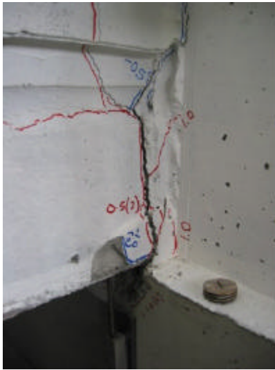
(a) Damage to the seat connection at 2.0% (1.95%) drift
