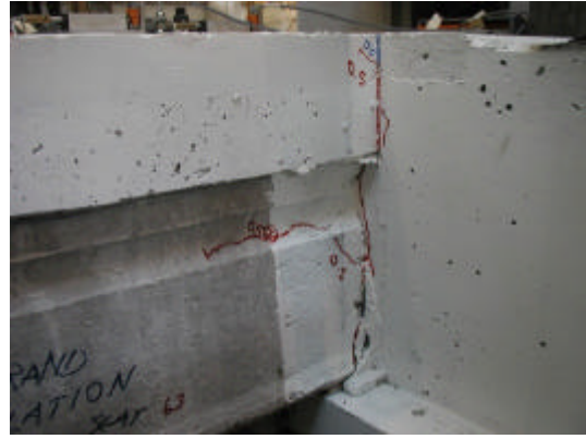
(b) Web split in the south face of the hollowcore unit.
