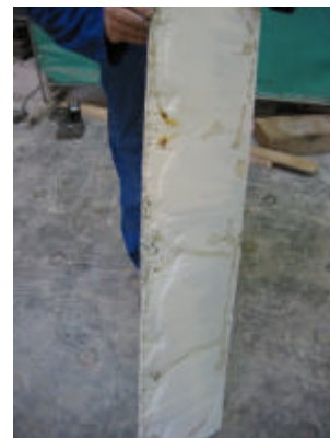
(b) Compressible backing board removed. Note indentations when it has been compressed.
