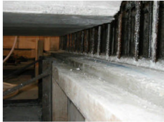
(b) Unit aligned just before the mortar bed is laid
