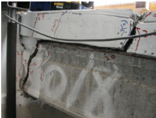
(a) The topping peeling away from the hollowcore unit
