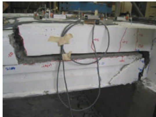
(b) Elevation of HC4 at the end of test
