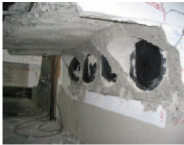
(e) The section of hollowcore unit attached to the beam (similar to the failure in the Matthews test)
