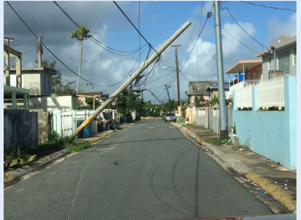
Author, Hurricane Maria, Puerto Rico, 2017
