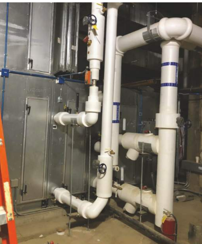
Rooftop pipe from building to cooling towers Pipe insulated with Foamglas & Metal Jacketing with Victaulic PVC Fitting Covers.
