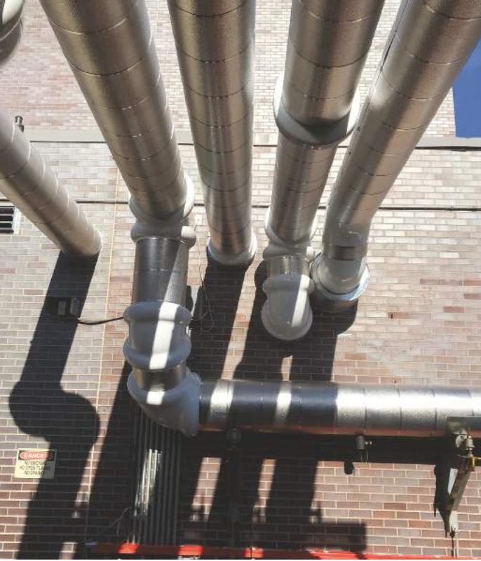
Rooftop pipe from building to cooling towers Pipe insulated with Foamglas & Metal Jacketing with Victaulic PVC Fitting Covers.
