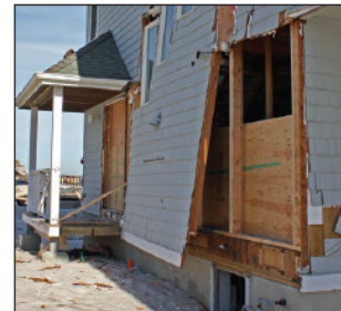
Figure 1: Back wall failure due to flood level above the lowest floor of a house in Ortley Beach, NJ.
