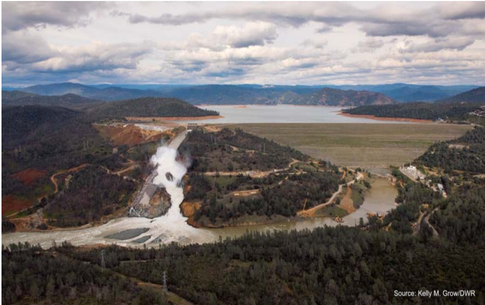
Oroville Dam Overtopping, 2017
