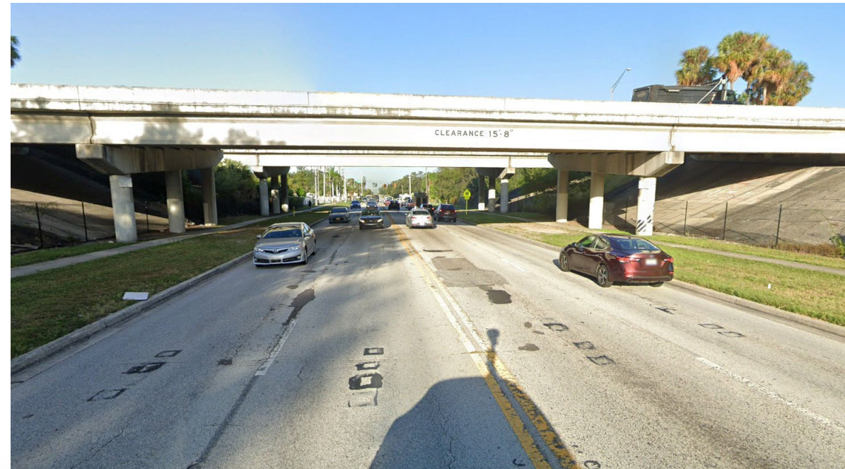
Existing bridge at 62 nd Ave N looking West
