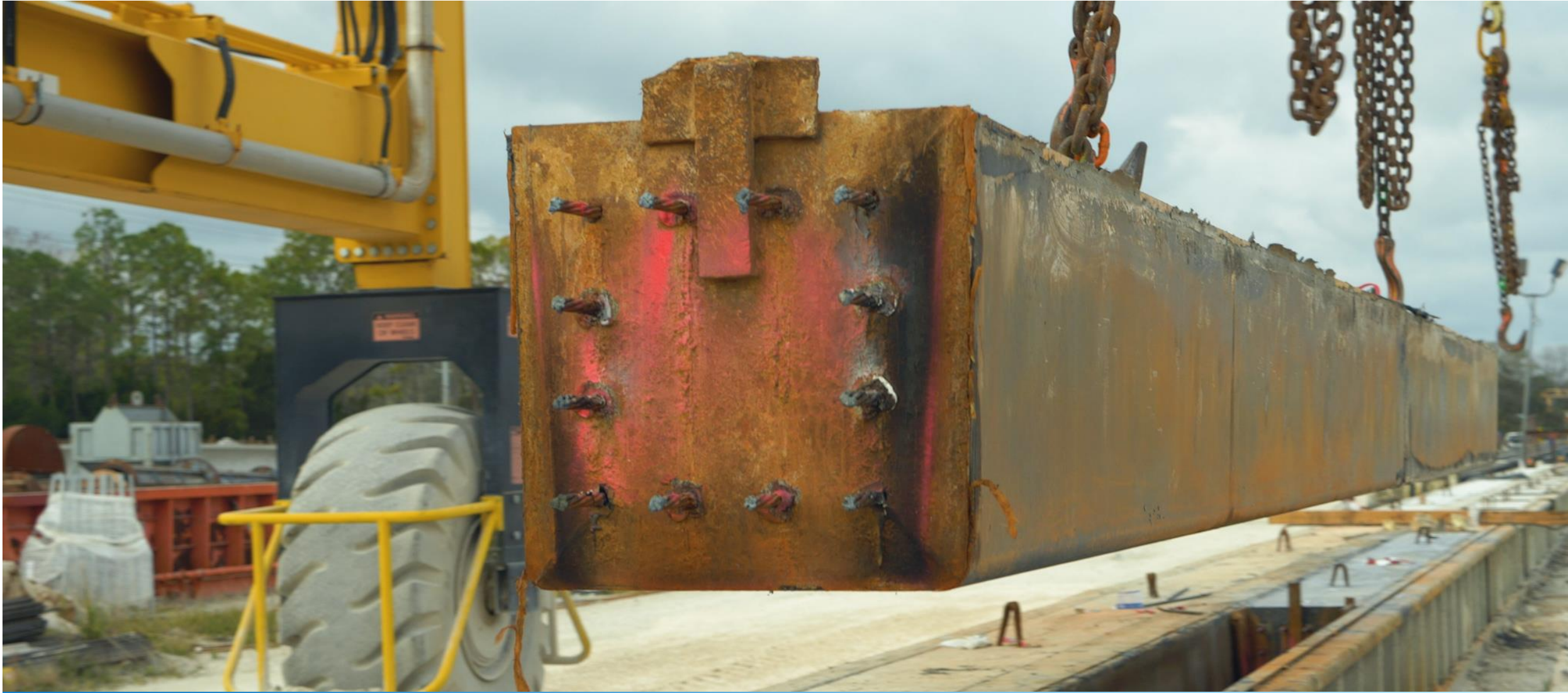
Pre-tensioned piling being removed from its form during Florida Dot tests at Dura Stress Inc.
