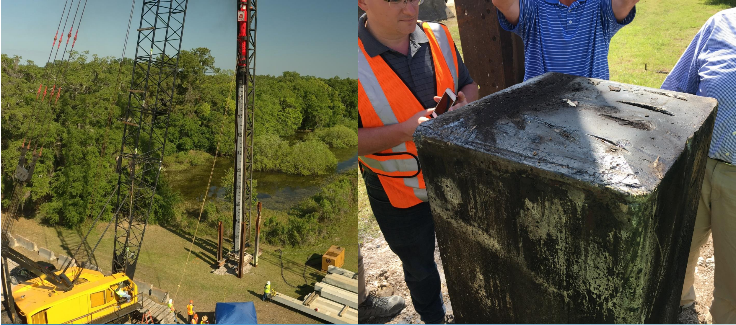
Installation of 18"x18"x100' square piling in Leware Construction Yard, Leesburg FL. Piling showed 100% integrity throughout installation.
