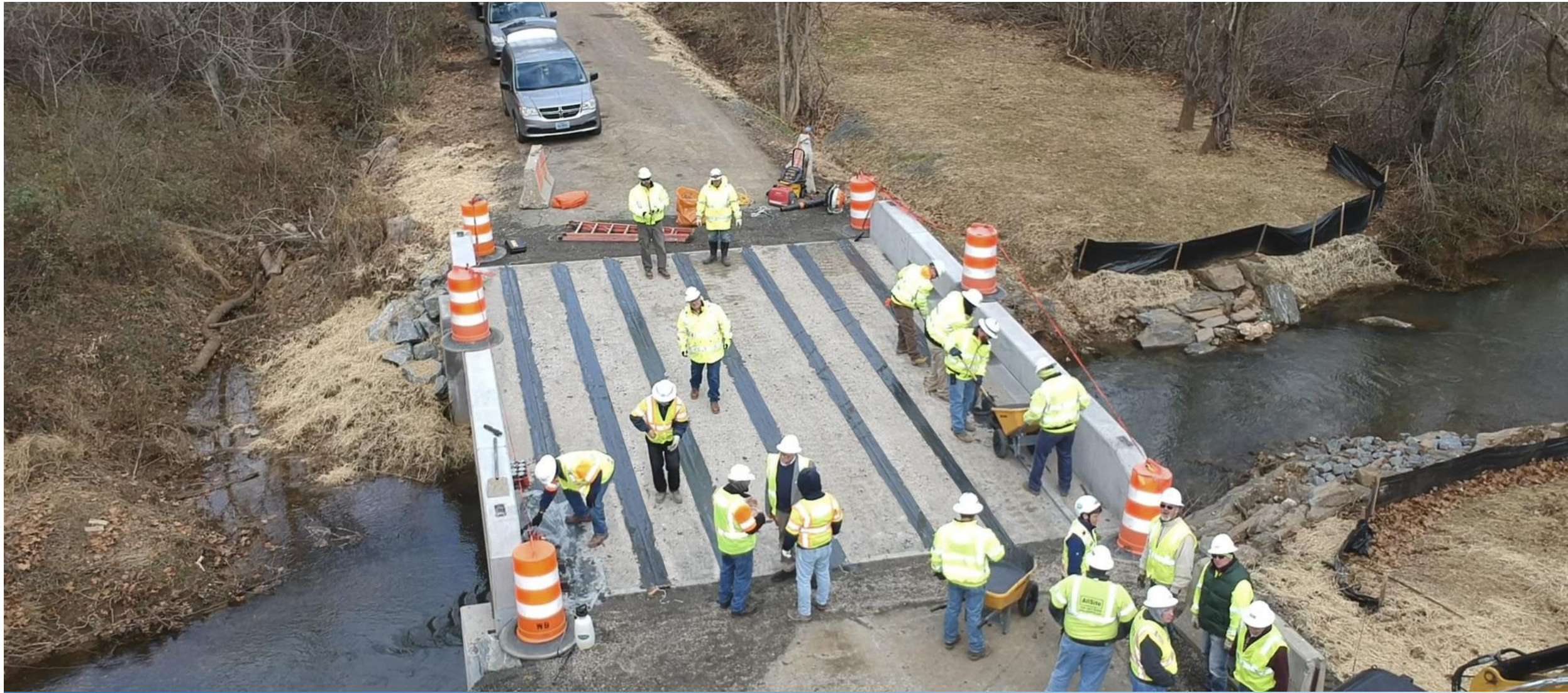
Aerial view of the VDOT crew pouring the bridge panel connections
