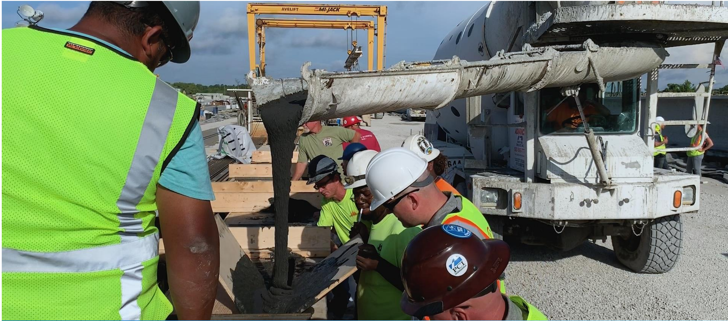
Cor-Tuf being poured via ready mix truck during H-piling casting at Dura Stress Inc.
