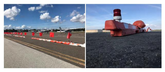
Use caution and avoid accidentally running over or tack-coating barricades during paving operations. Barricades will be connected or spaced at a <u>maximum of 4 feet</u>. Barricade Flags are supplemental and as directed by the owner. Barricade Lights will
