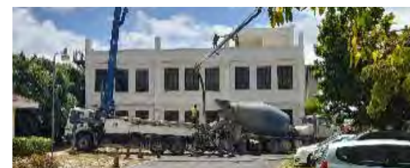
Renovations ongoing at Secretariat Building
