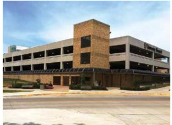
The University of Missouri Health Care Patient and Visitor Parking Structure (referred to as the MUHC Garage) was built in 1986 with a capacity of 448 vehicles. The MUHC Garage consists of three elevated post-tensioned (PT) concrete decks and a slab-on-ground.
