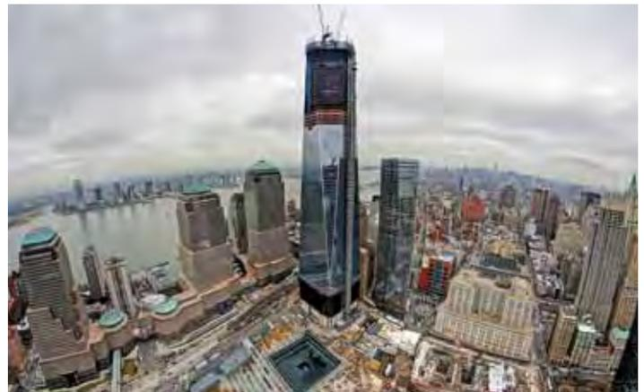
**Construction of One World Trade Center in Lower Manhattan, New York City, USA, uses 45,000 U.S. tons of high-strength structural steel. At 1,760 feet tall, the 104-floor superstructure will now be the tallest building in the Western Hemisphere. © Photo courtesy of The Port Authority of New York & New Jersey. Used with permission.**
