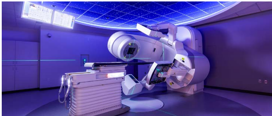
Recent work for Oregon Urology Institute featuring a precisely engineered concrete vault built to safely contain radiation from their new linear accelerator.
