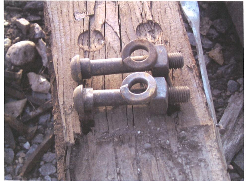
Figure 3-19 1" x 6" Oval Necked Track Bolts – Photo by J. E. Riley
