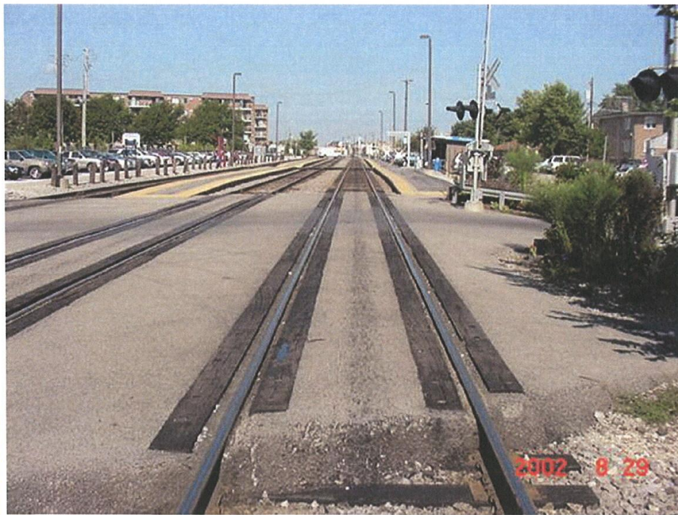
Figure 3-66 Asphalt & Timber Flangeway Crossing - Photo by Robert Schuster
