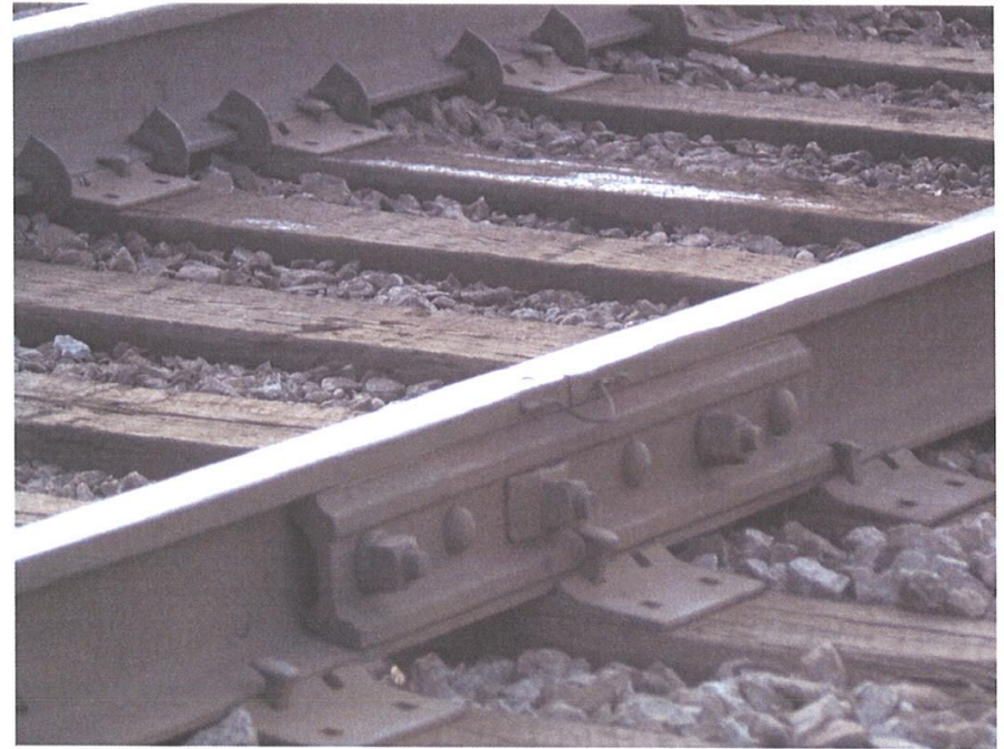
Figure 3-9 Standard Head-Free Joint Bar – Photo by J. E. Riley
