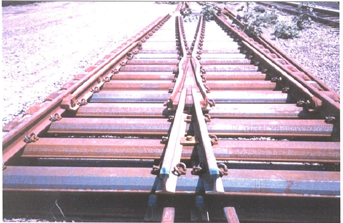
Figure 3-6 Steel Ties
