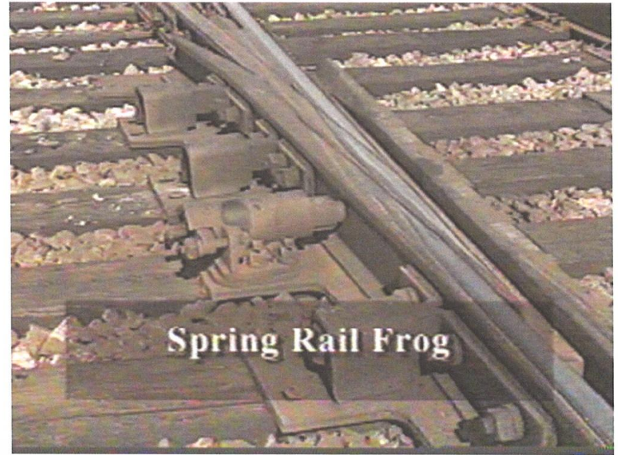
Figure 3-34 Spring Frog - Courtesy of the Union Pacific Railroad
