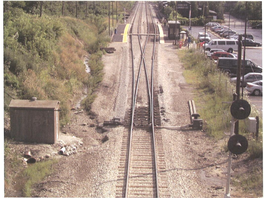
Figure 3-26 Equilateral Turnout - Photo by J. E. Riley
