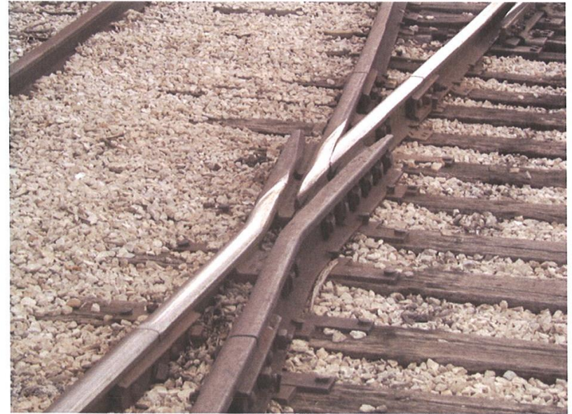
Figure 3-36 Bolted Rigid Frog - Photo by J. E. Riley
