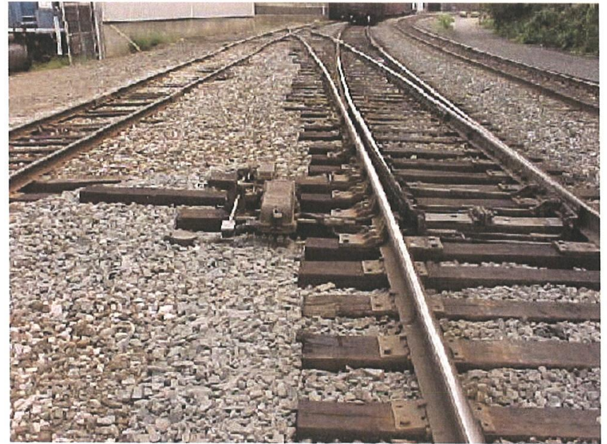
Figure 3-3 Switch Timber – Photo by Craig Kerner
