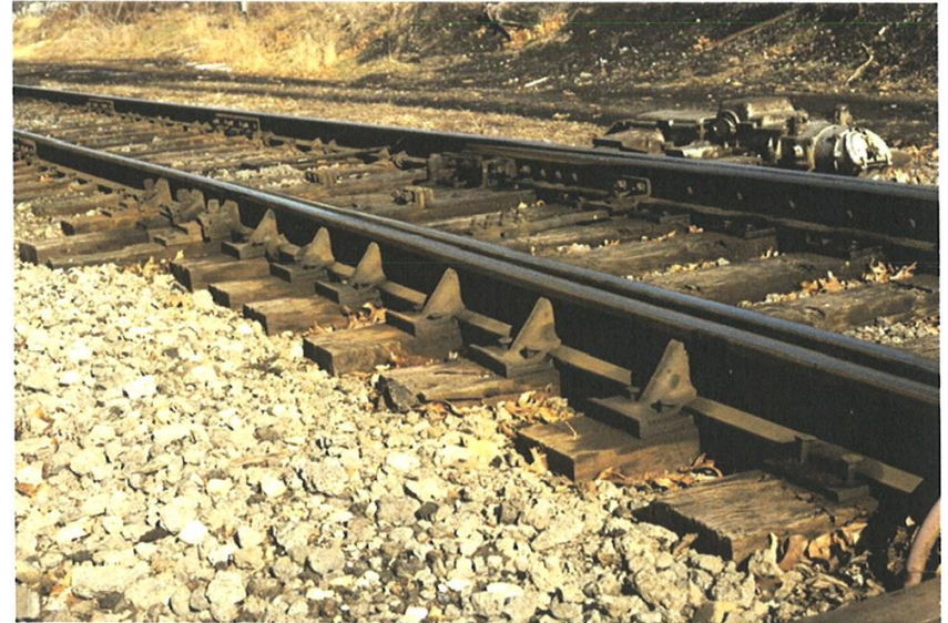
Figure 3-52 Rigid Type Rail Braces
