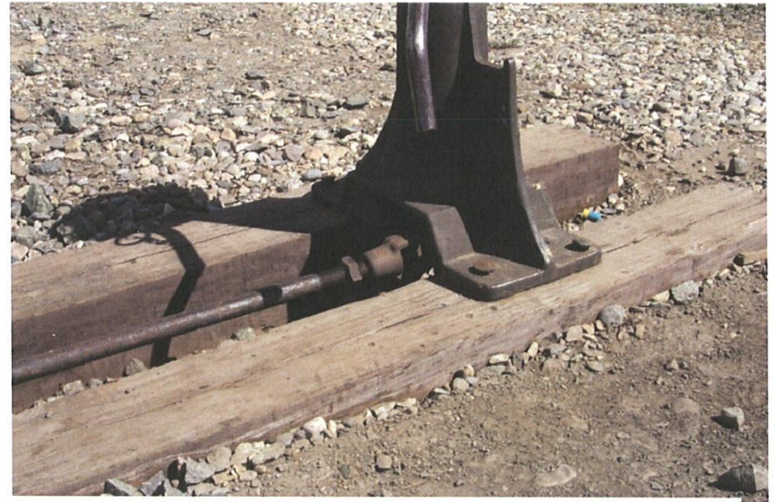
Figure 3-38 Head Block Ties
