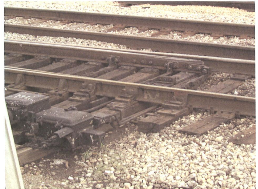
Figure 3-60 Dual Control Power Switch - Photo by J. E. Riley
