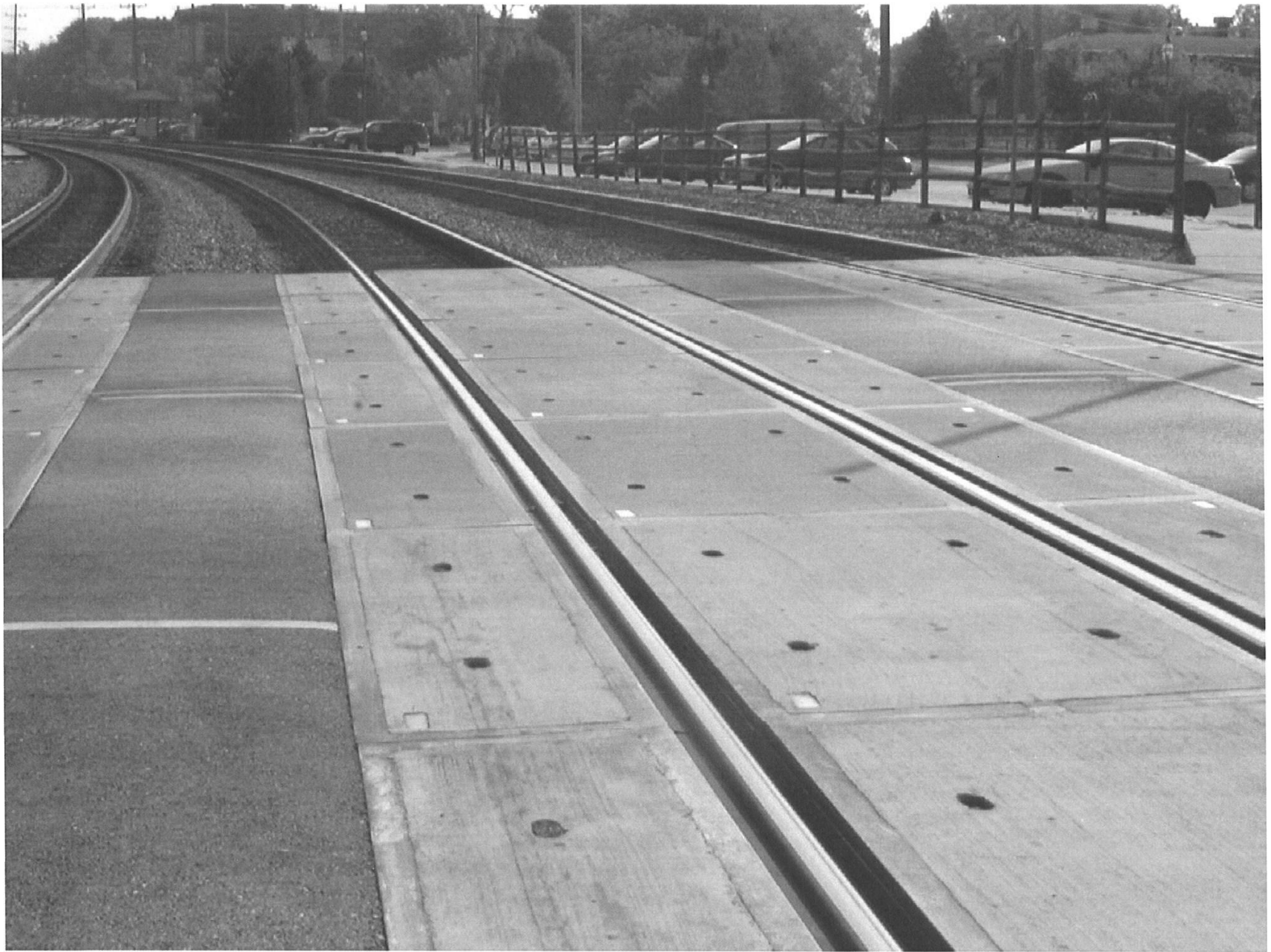
Figure 3-67 Precast Concrete Crossing - Photo by J. E. Riley
