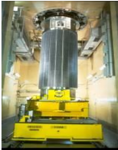
Wet or dry unloading at La Hague
