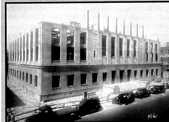
The Mobile courthouse under construction in April 1935. (National Archives at Atlanta)
