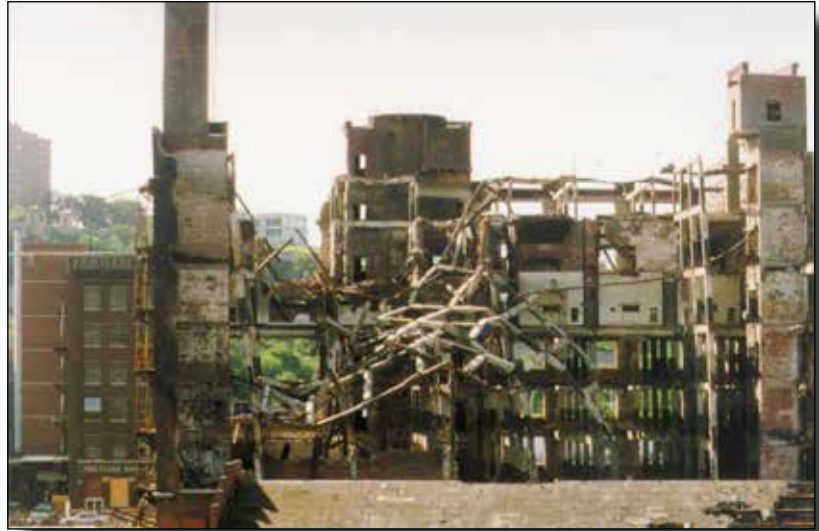
The seven-story Sunshine Biscuit building was destroyed in a major fire in 1998, and came into Brownfields / Voluntary Cleanup Program in 2000.
