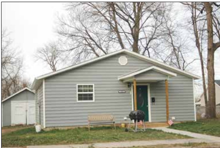
A condemned house (top) was rebuilt. Police found that as problems were fixed, the neighborhood started to improve dramatically, both in appearance and lowered crime rates.
