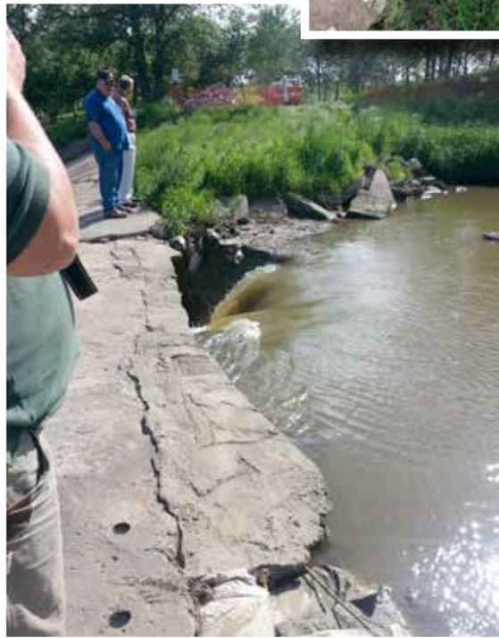
Resources (MDNR). There was no immediate danger of breach, stated MDNR experts, yet they recommended filling the hole with riprap as a temporary measure to slow the water down. With that accomplished, they turned to the consulting engineers for recommendations for a more permanent repair.
