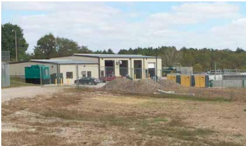
**The operations of the Richmond sewer plant are consolidated at one location, including the control center, lab, maintenance area and storage.**
