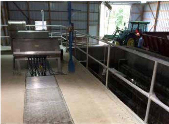
The effluent (water) that leaves the treatment passes over several banks of ultraviolet lights, in order to kill any remaining bacteria that have not been removed through the processing by the plant's sequencing batch reactor.
