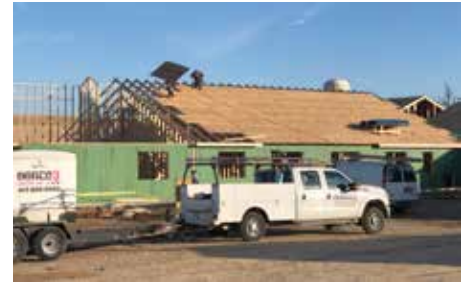
Senior Living and Memory Care Facility
