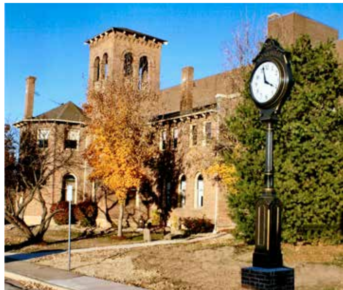
Top: The downtown square in Waynesville needed repairs. Moss grew on the facades of buildings; a tree grew through another building; and there were many empty storefronts. Photo by Alan Clark
