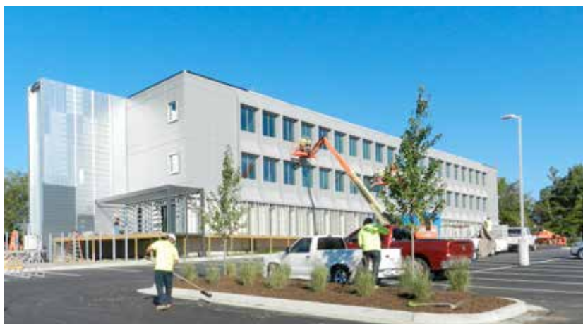
Top: LEED buildings strive to have a minimal impact on the environment. Twenty percent of the materials used are recycled. Wood from an old barn in Kentucky was reclaimed and used for key design features throughout the building. Above: The Center was designed to bring in the natural light from outside, by allowing the light from the large perimeter windows and adding glass walls to office walls that would customarily have been drywalled.
