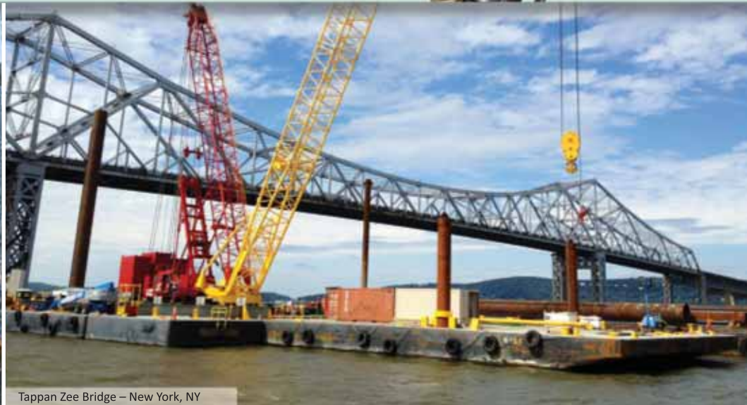
Tappan Zee Bridge – New York, NY
