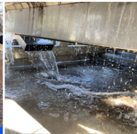
(a) TWAS gravity belt (b) Dewatering (c) Dewatered TWAS cake solids (d) Combined filtrate and wash water flowing into sump.
