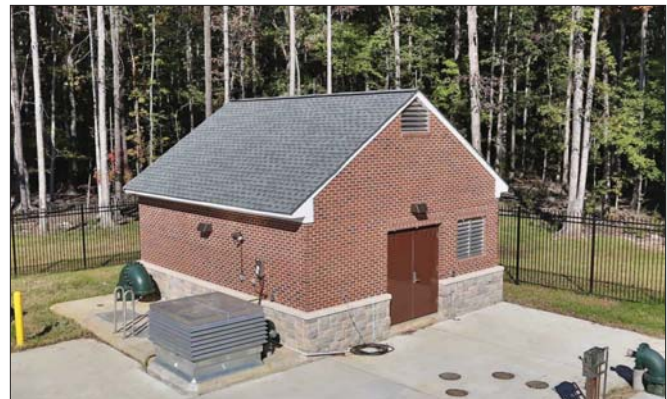
Oyster Point Tech Center Pump Station | City of Newport News, VA
