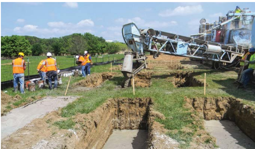
A construction crew installs a 108-by-108-by-84-in. tee to connect two pipelines.
