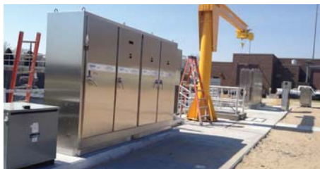
New UV System Retrofit
