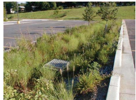
Examples of bioretention
