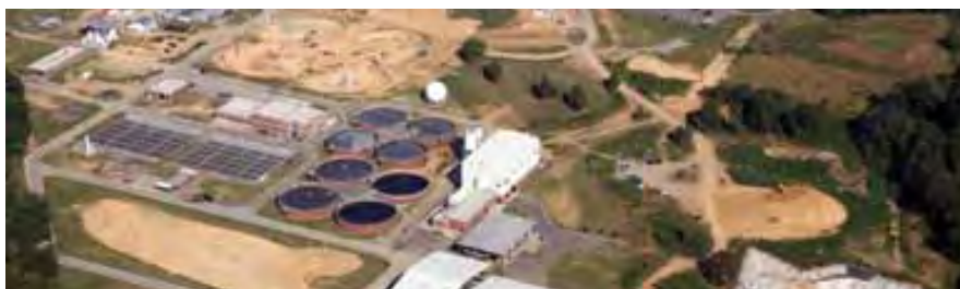
Aerial photo during headworks and primary treatment construction
