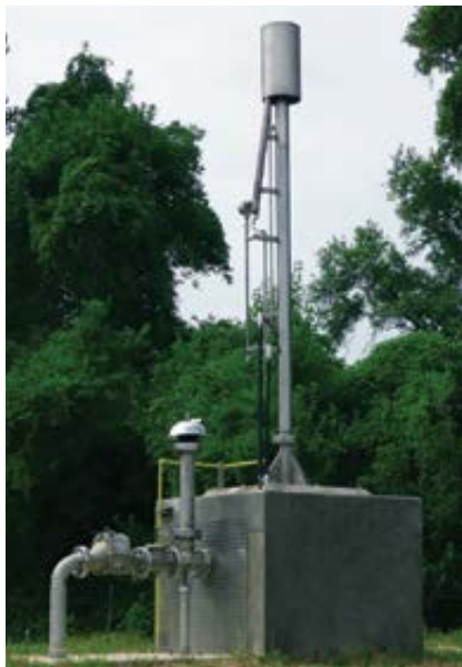
Candlestick Waste Gas Flare with Remote Tip Ignition
