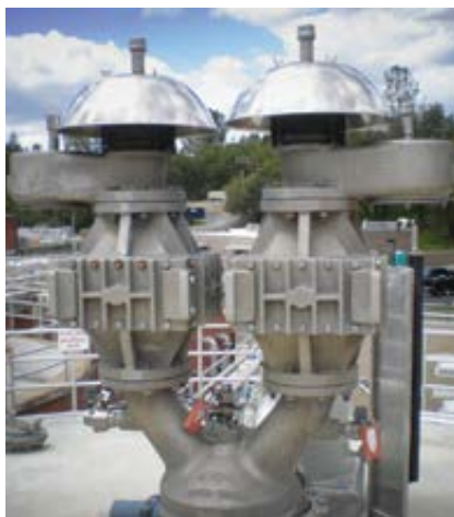
3-Way Safety Selector Valve with Combination Flame Arrester and Conservation Vent Units
