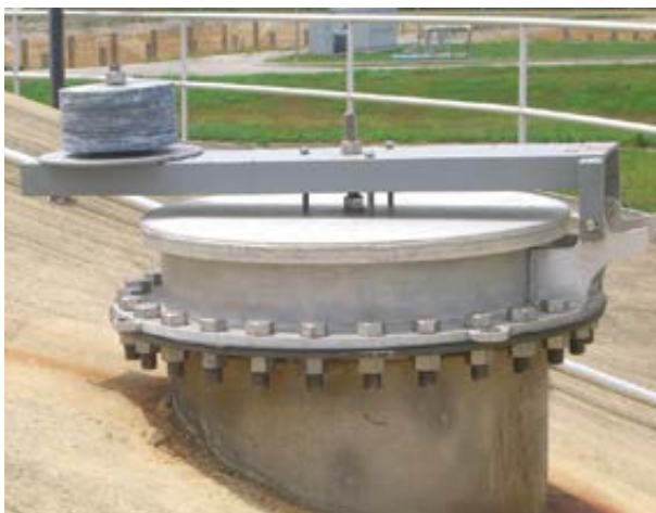
Weight Loaded Emergency Vent/Manhole Cover
