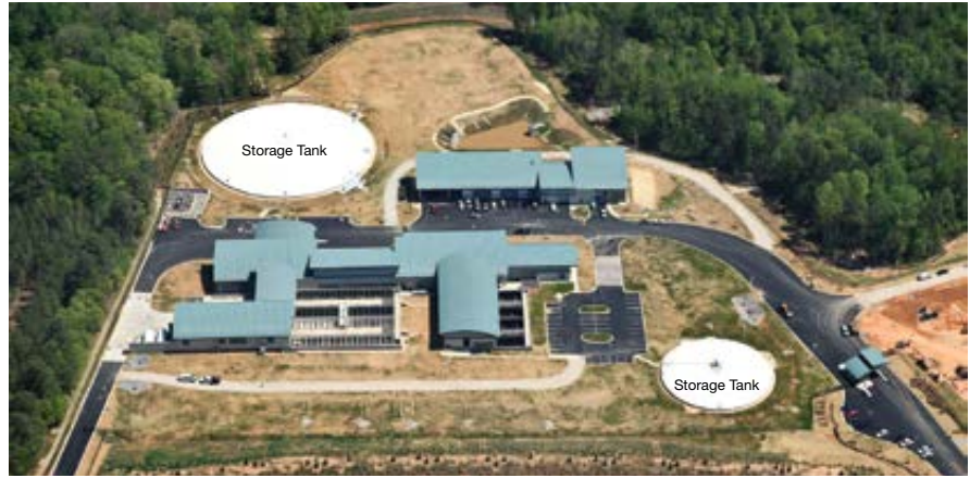
Figure 1 – Aerial view of the D.E. Benton WTP showing the storage tanks painted with a high albedo paint to reduce the heat island effect.
