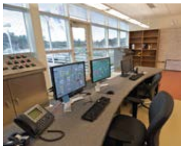
Figure 2 – View from the D. E. Benton WTP Control Room.
