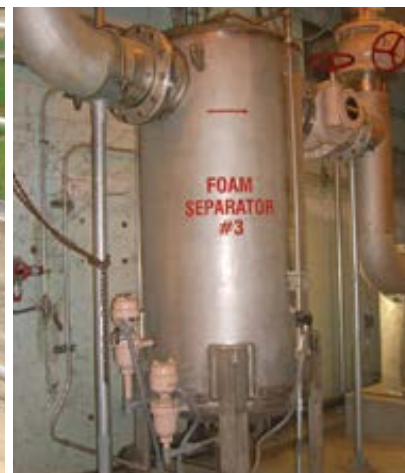
Foam Separator with High and Low Level Switches
