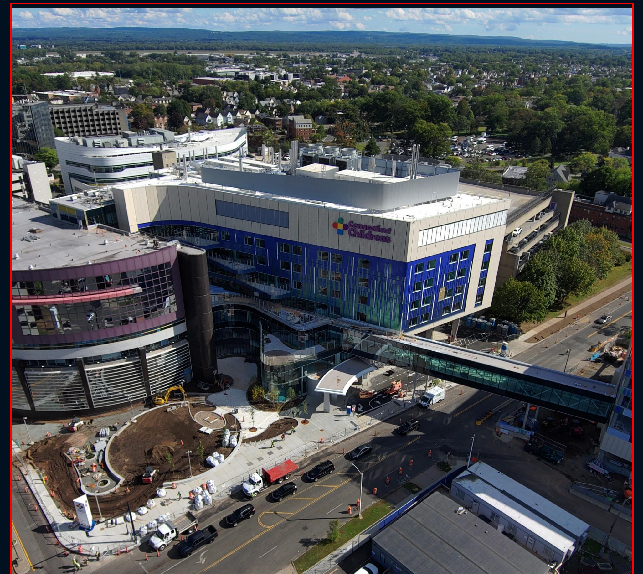
Connecticut Children's – NICU Tower Expansion Hartford, Connecticut
