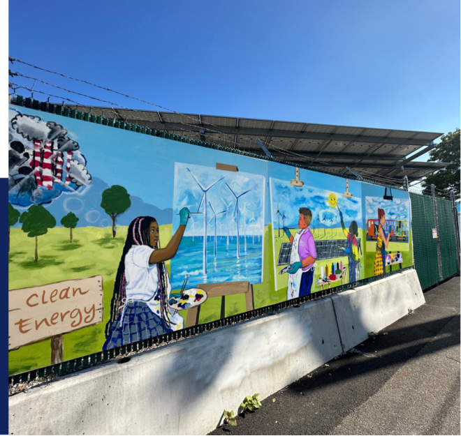
Elementary student mural outside a 3 MW energy storage installation providing grid services to the Pelham Gardens neighborhood of the Bronx (courtesy of NineDot Energy).
