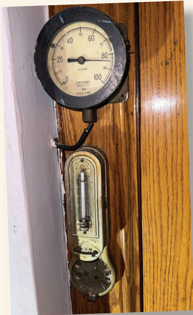
Image of an old thermostat, submitted by Aryeh Kaplan, AK and Sons Plumbing Corp.
