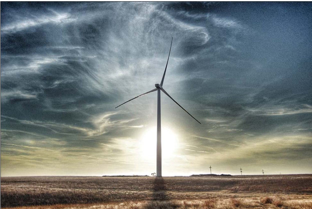
The sun goes down over the second turbine fully erected at the east edge of the Osage Wind project.
