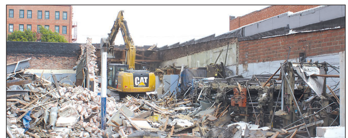
Signage is removed from the Sapulpa Herald (top) before the building is demolished (below).
