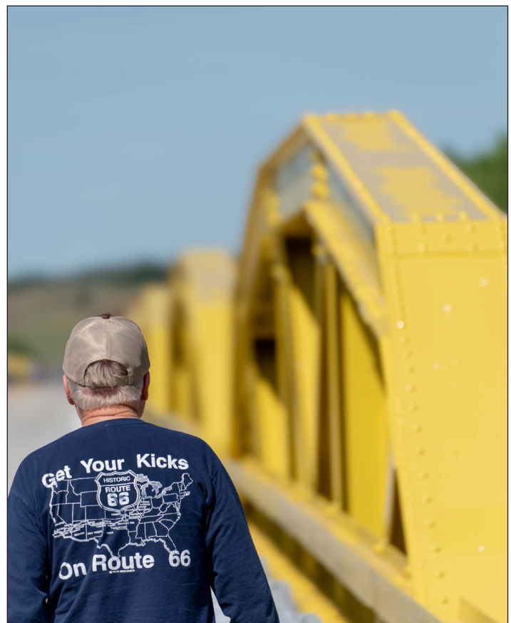
Before the reopening of the iconic Rt. 66 Pony Bridge to the vehicle, the longest truss bridge in Oklahoma and on Rt. 66, visitors and locals could walk the length of the historic structure.
