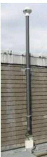
Antennas should be mounted lower than the building lightning conductor and directly connected to an approved ground point. Lightning arrestor technology should be fitted to points of entry and exit to and from the building. Any external distribution boxes and lightning protection enclosures should be rated to at least IP66. These photographs show the devastating effect of poor grounding and poorly installed equipment. The antenna
