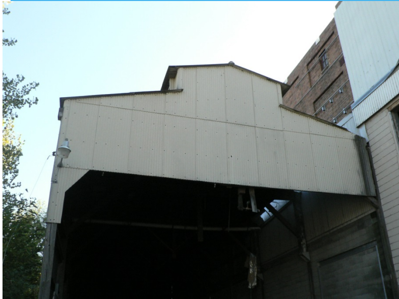
Corrugated Asbestos-Cement Sheets
