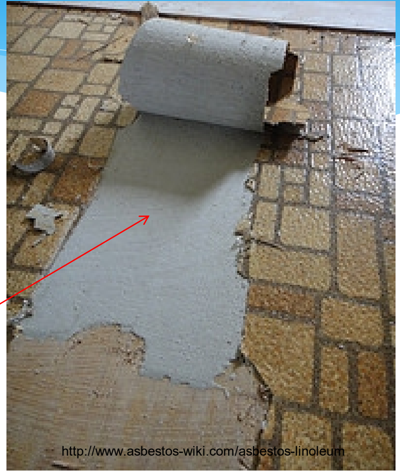
Vinyl Sheet Flooring/Linoleum
