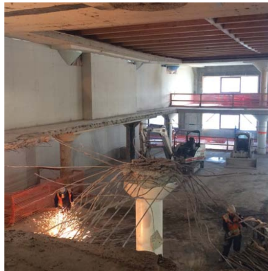
Removal of floorplate and columns
