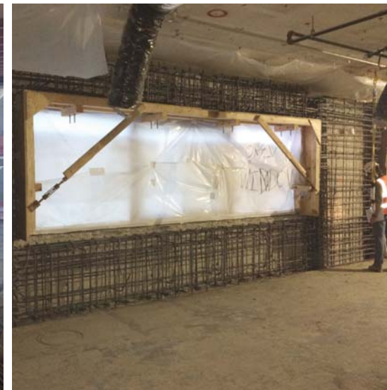
Rebar along exterior shotcrete wall
