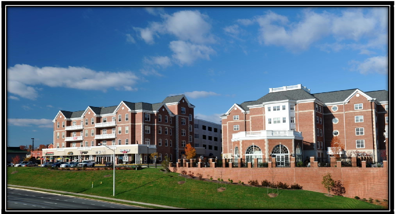
Eagle Village Mixed Use Development – Phase I – Opened 2010
