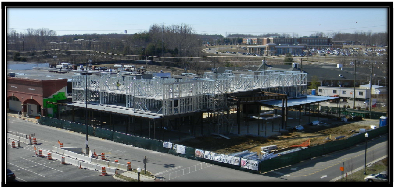
Hyatt Place – Fredericksburg – Construction – February 2013
