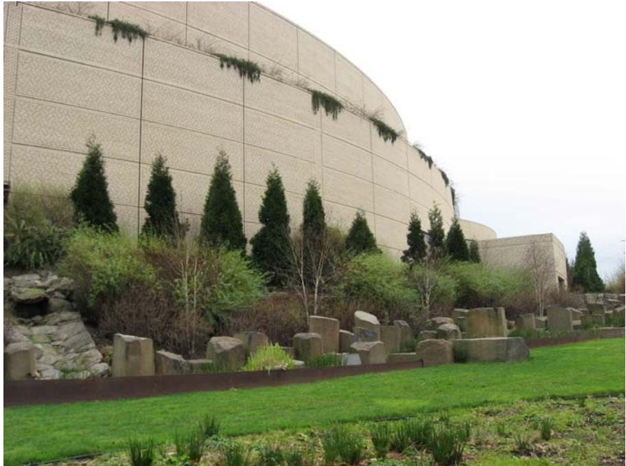
The Oregon Convention Center saves $15,600 annually on its stormwater bill by managing roof runoff in rain gardens along the side of the building.
