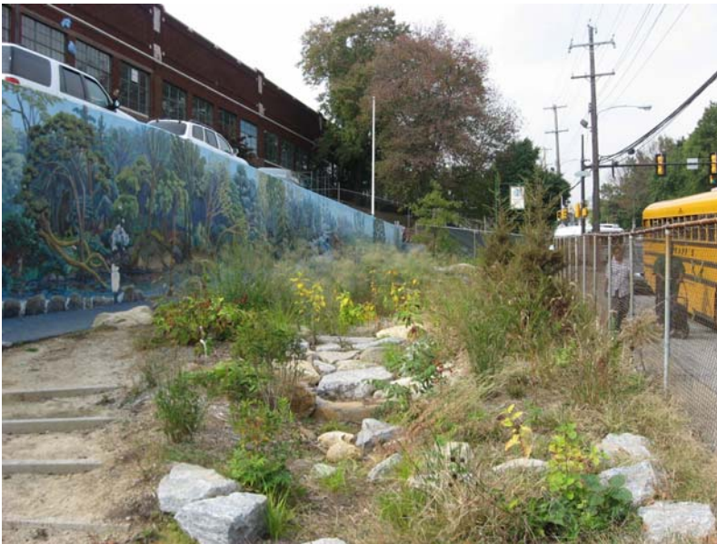
Philadelphia's new impervious-based fee encourages retrofits of large impervious sites, such as the Wissahickon Charter School (above), which now intercepts all parking lot runoff with rain gardens.
