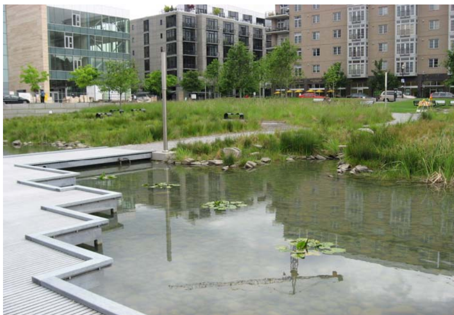
Tanner Springs Park in Portland, Oregon includes a constructed wetland for managing runoff from nearby buildings
