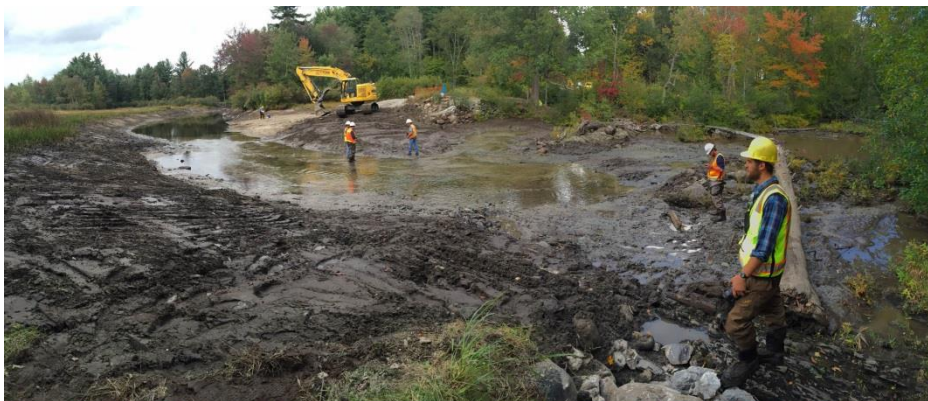
Removal of this dilapidated dam reconnects 40 upstream river miles on a beautiful trout stream in Pepperell, MA. Removal was completed in 2015.
