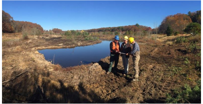
Currently under construction, the Tidmarsh Farms Restoration project will restore approximately 3.5 miles of stream and 250 acres of wetlands in Plymouth, MA.
