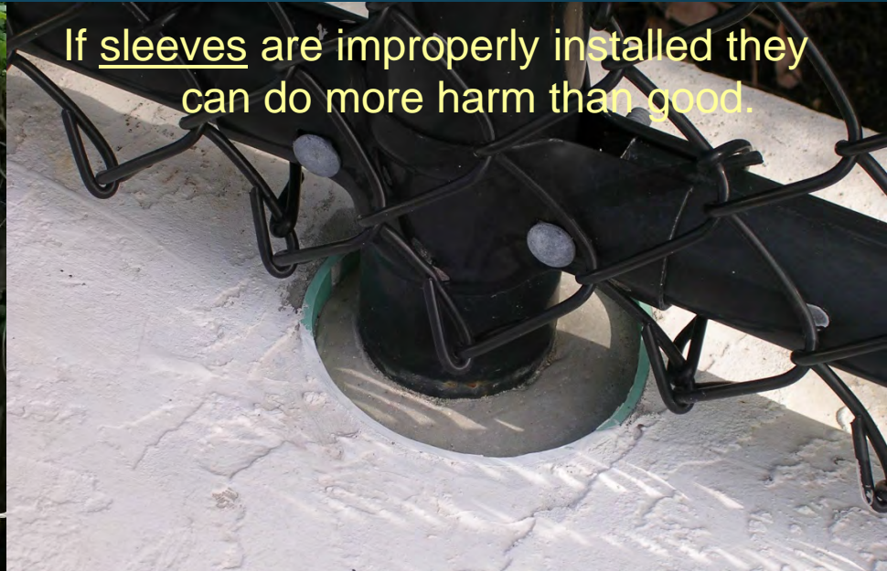
Sleeves can be surface-mounted when you cannot go deep.
