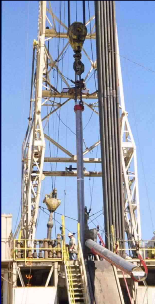
16in titanium alloy casing being installed
