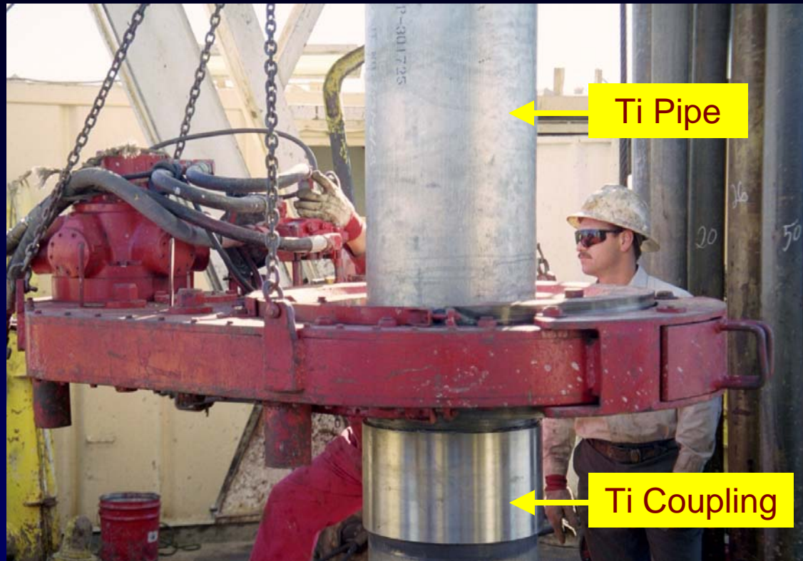
16in titanium alloy casing being installed
