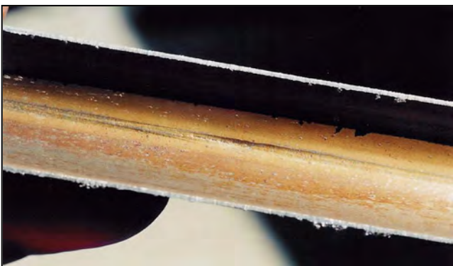
Figure 8 Tube Section Suspect Weld Deformity
