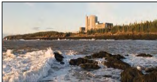
Figure 4 Point Lepreau Nuclear Station
