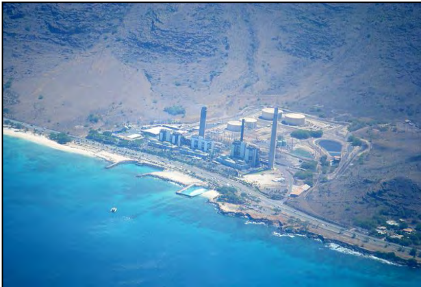
Figure 7 Kahe Unit 1 Generating Station
