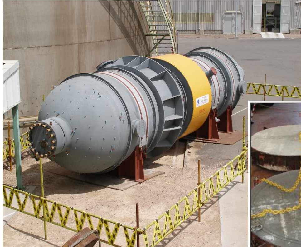
SNAMPROGHETTI Zirconium Urea Stripper - Courtesy of Luigi Resta
