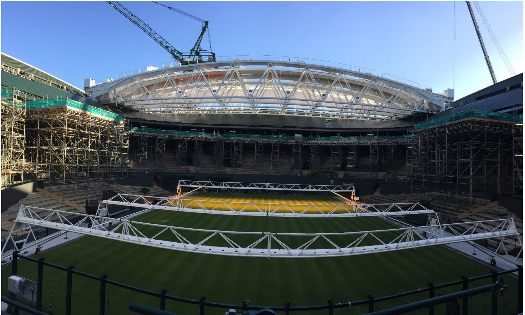
Wimbledon No1 Court Roof
